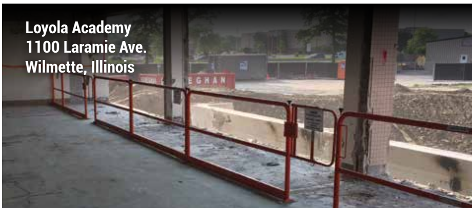
The 'old way' (2x4 railing to the right) The 'new way' Switch Rail System to the left
