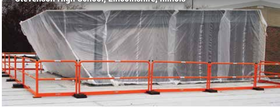
Counterweight System on EPDM Roof Stevenson High School, Lincolnshire, Illinois
